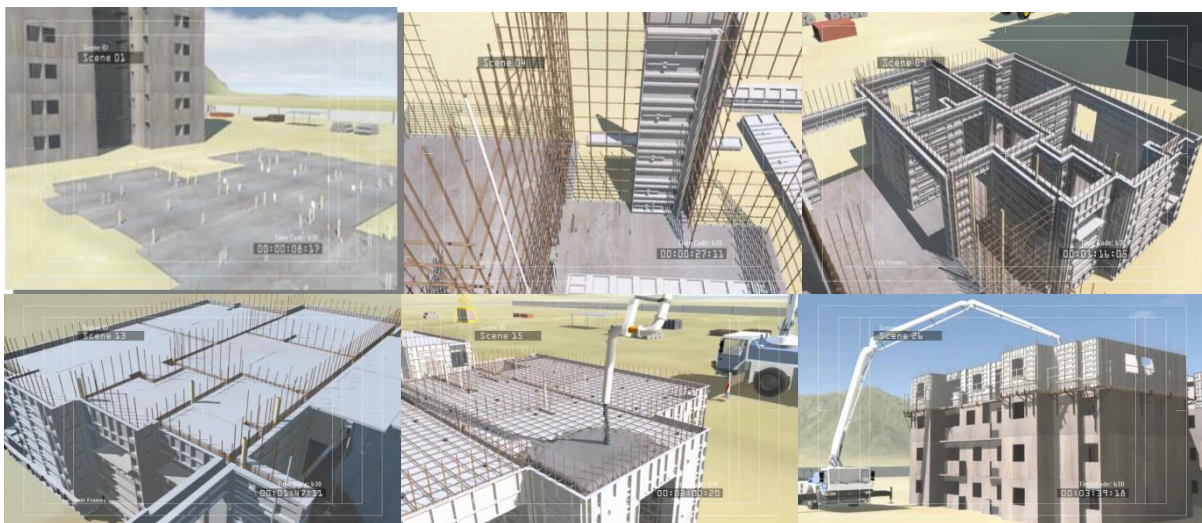
Fig. 10–Structure implementation stages, Showing Concrete Walls Arrangement.
